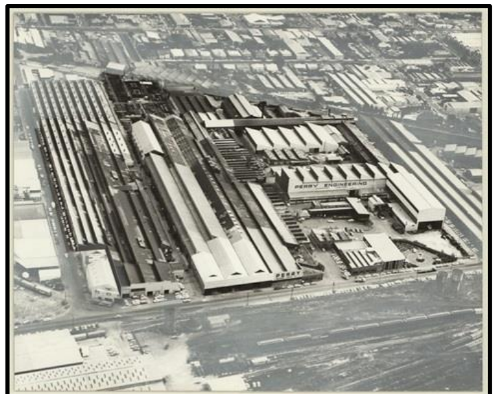
Perry Engineering Mile End South [westtorrens.sa.gov.au]
