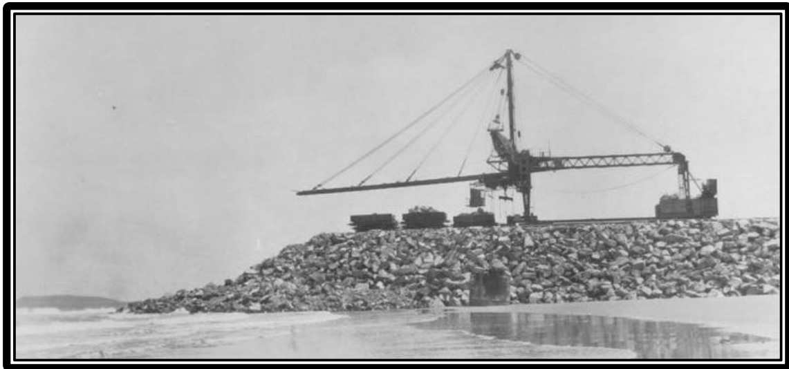
1935 The Telfer crane constructing the southern breakwall. NQBP Collection
