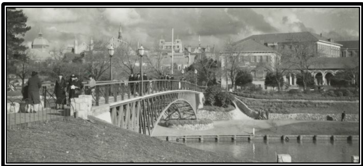
Circa 1937 University Footbridge B 35481 State Library of South Australia
