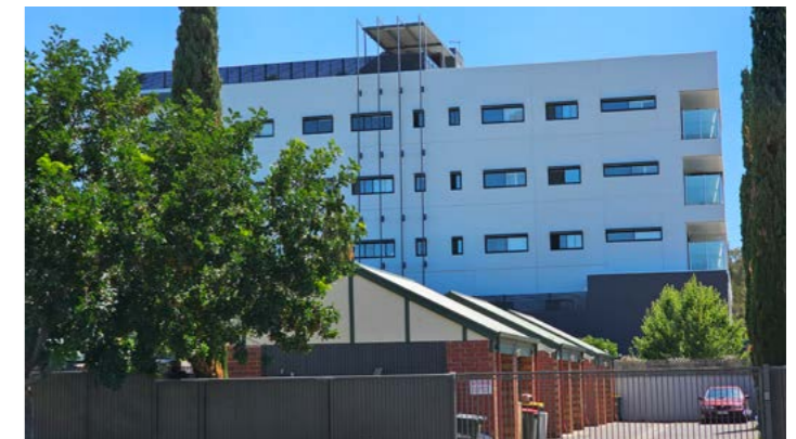
Example of 5 storey apartment development that lacks articulation in its built form and causes overlooking issues to adjoining neighbours.
