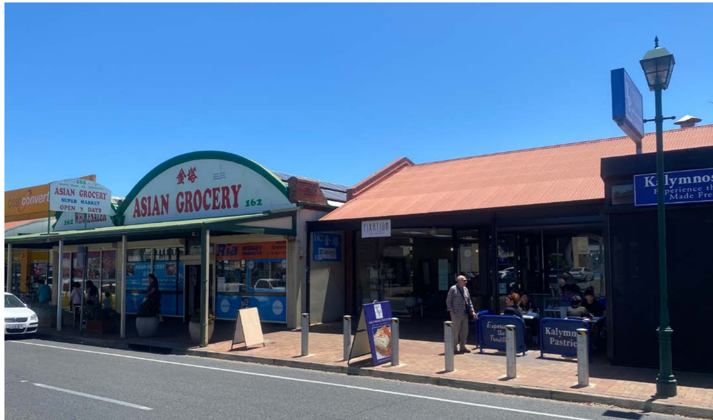
North side of HB Rd on the corner of Shipster St.
