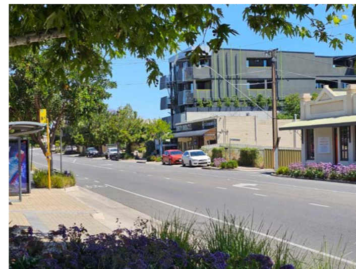
5. Urban corridors grow over time. Investment into the public realm is usually a catalyst that attracts more private mixed use development.
