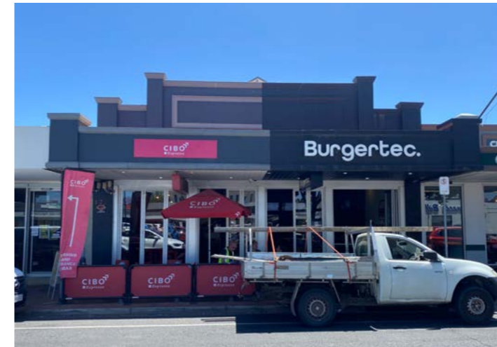
The dimensions of the road and presence of verandahs pose a challenge to increasing canopy cover on the north.
