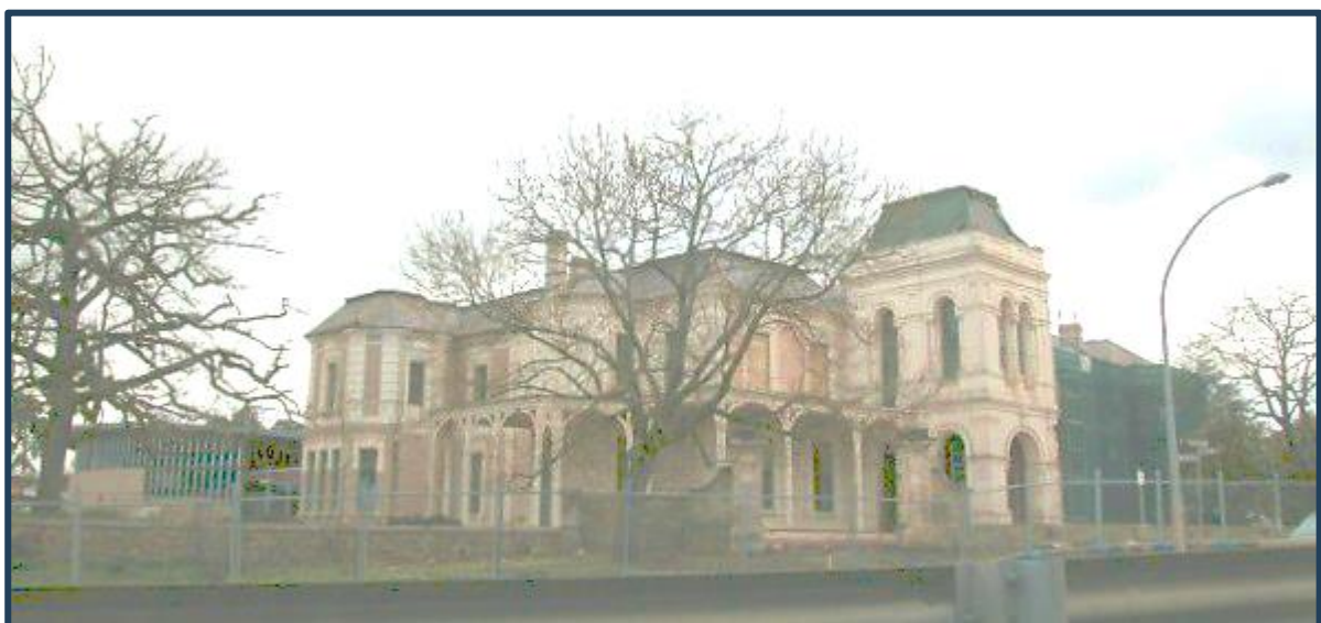
Auchendarroch before restoration, Mount Barker Heritage Survey, 2004
