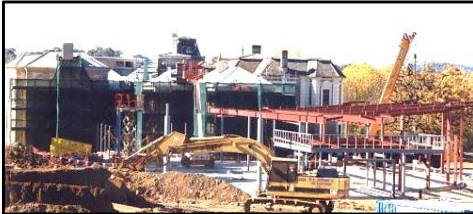
Auchendarroch and Wallis Tavern redevelopment, May 2002, [MBHS PH-V50-00013]
