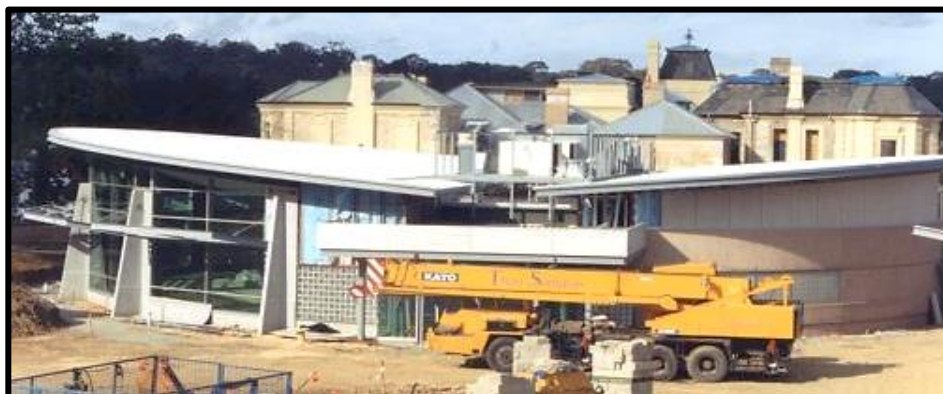
Auchendarroch and Wallis Tavern redevelopment, May 2002, [MBHS PH-V50-00036]
