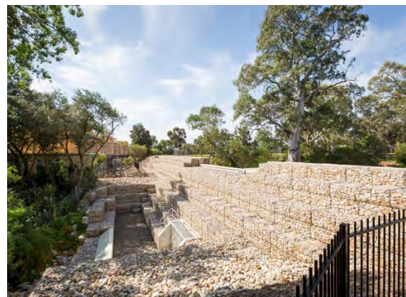
Flood Control Dam
