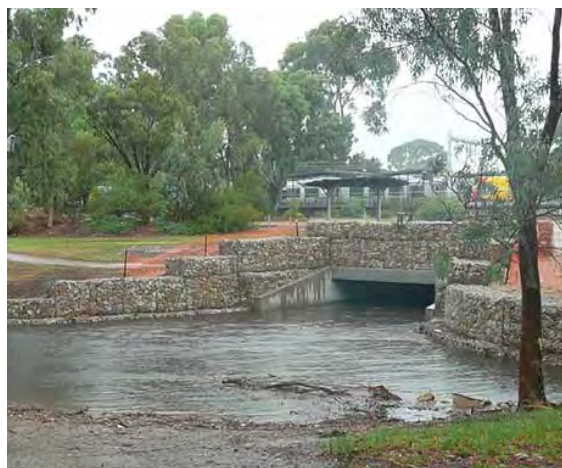
Constructed Culvert
