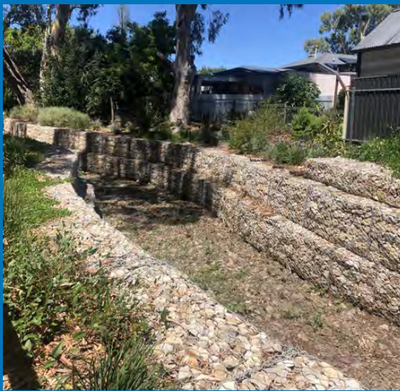
Rock filled gabions
